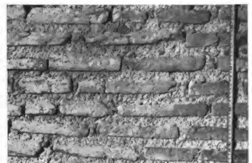
Fig. 89d. S. Martino ai Monti, Roman Hall, brickwork c; south façade of vaulted Hall after rebuilding
